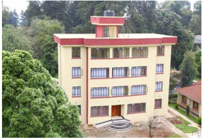
The new ultra-modern SOTERIA TRAINING WING constructed to increase the facility's training capacity
